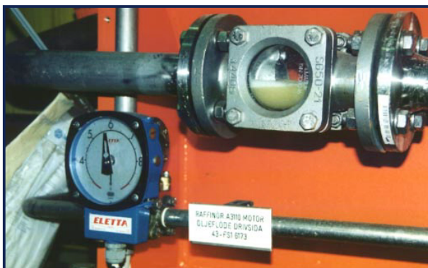
The differential pressure principle, well suited for measuring flows of both oil and water
