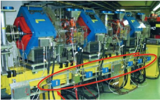
CERN, France. Magnets that are under high voltage focus the particle beams. Eletta flow Monitors control the cooling circuits.
