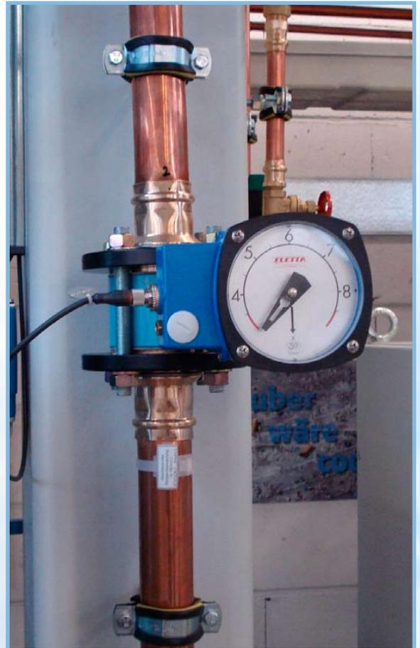
*Eletta flow meters in induction heating systems from EFD Induction.*
