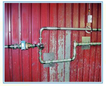
An SP-GA flow switch mounted horizontally. Eletta flow switches work independently of their position which is one of their advantages.
