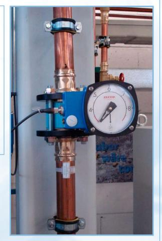
Eletta flow meters in induction heating systems from EFD Induction.
