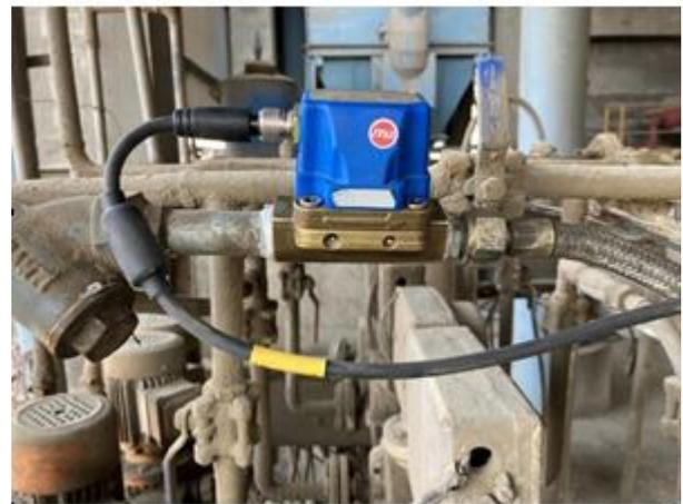
Now end user team is looking for confirmation from Grinding aid chemical supplier on it's suitability with Brass & Nitrile rubber parts so that we can use the economical version of Eletta M Series flow meter.
