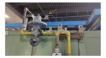
For a glass bottle manufacturing unit, Eletta has supplied a complete solution of 8 units of M Series flowmeters in 1" threaded connections, M310-G25SS, for the 8 different lines of burners of LPG gas measuring a flow range of 6.5-to-65 Nm3/h. And a 4" wafer connection, M310-F100SS for 60-to-600 Nm3/h of LPG flowing through the main header line from the storage tanks to these 8 burner lines.
