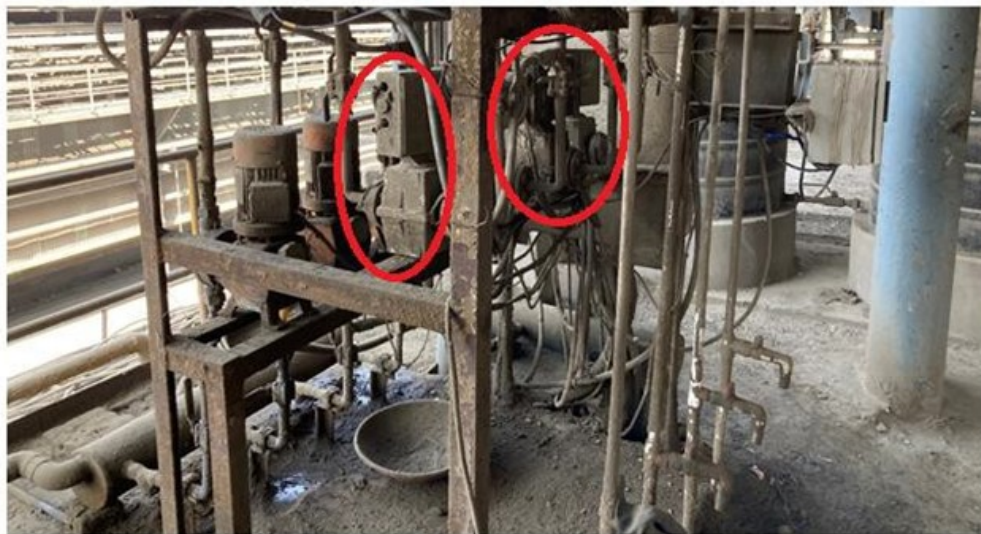
Red circle shows existing ABB Make Electromagnetic flow meter in grinding aid chemical dispensing skid at Ambuje Roper plant
